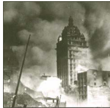
Fire engulfs the Call Building
