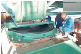
A F.P. installed as part of a seismic retrofit of the Hernando DeSoto Bridge in Memphis, TN.
